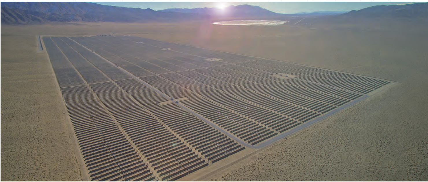
65 MWp photovoltaic power plant in Luning, Nevada, USA, 2016 built by order of Invenegy Solar Development LLC
